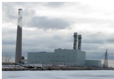
Portland Energy Centre
